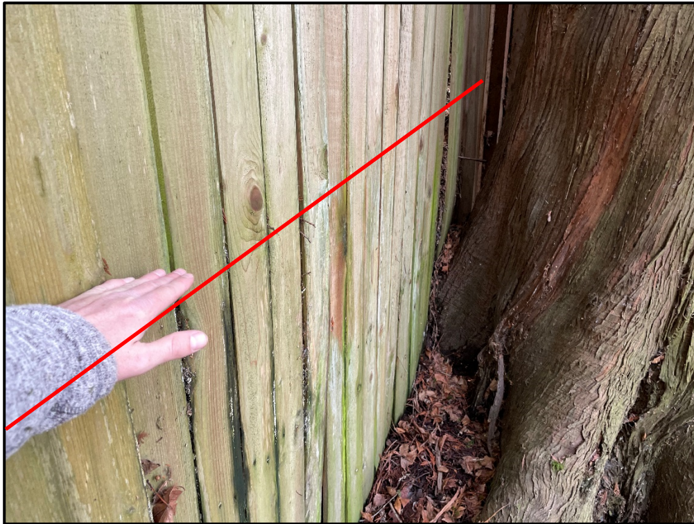
Photograph 3. The base of tree 219 in relation to the fence on the southern property line. The red line indicates the approximate level of fill against the fence to the south.
