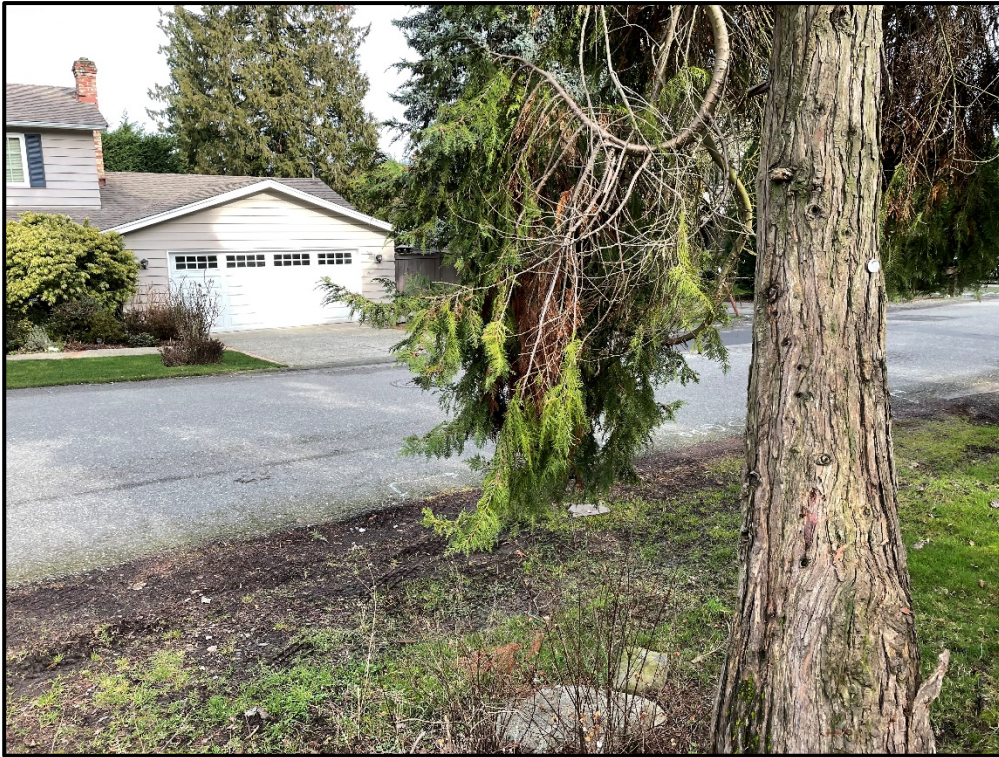
Photograph 7. Photo of tree 226 taken in the direction of the lower trunk lean. The tree targets immediately to the right of the garage in the photo. Three phase power lines are immediately out of frame above the photo.
