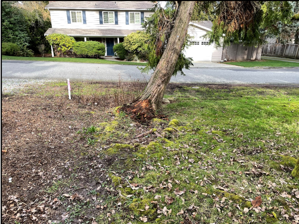
Photograph 6. The base of tree 226 showing the swept base and lower trunk lean.
